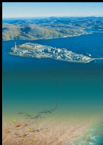
TERMINAL: The plant at Melkøya in northern Norway became operational in 2007.
